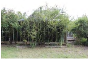
I4 veranda facing S
