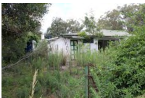
O2 House Facing NW
