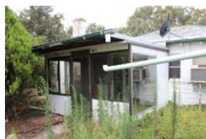
South Elevation Sunroom Facing N
