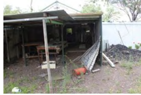
M2 Shed Facing W
