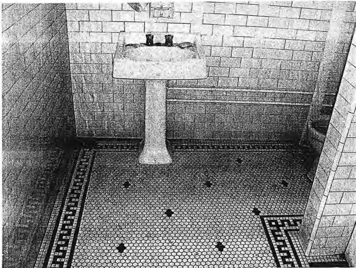
Central Bathroom - Floor & Wall Tiles & Sanitary Fittings
