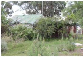
N1 Shed facing NW
