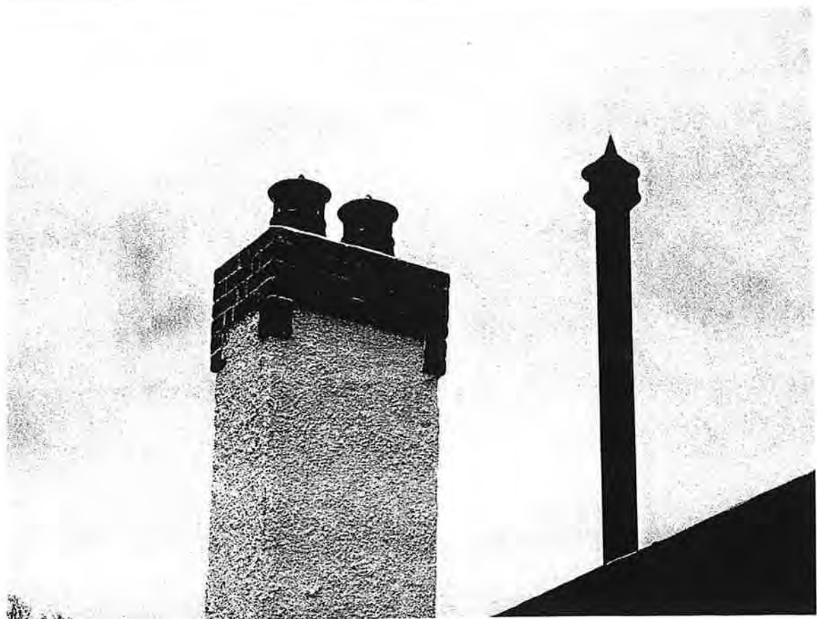
Chimney Detail & Vent Pipe (with cast cap)
