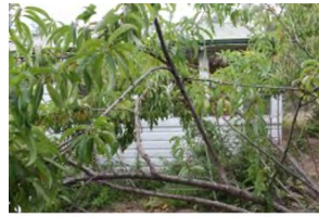
Toilet South Elevation Facing N
