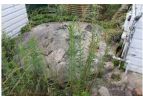
P2 Tank Pad Facing N
