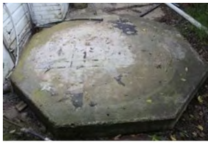
T1 Tank Pad Facing S
