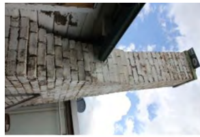
T2 Chimney Detail Facing SE
