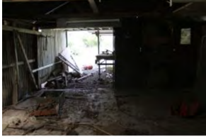
L1 Shed Ground
