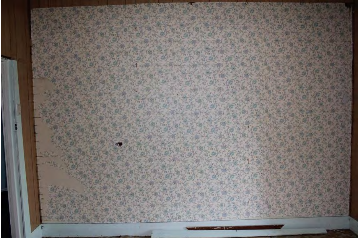
Photo 9: Internal original wall (bedroom 2) showing wallpaper and weatherboard construction
