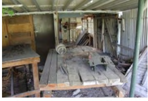
K1 Shed Facing NW
