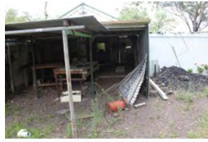
M2 Shed Facing W
