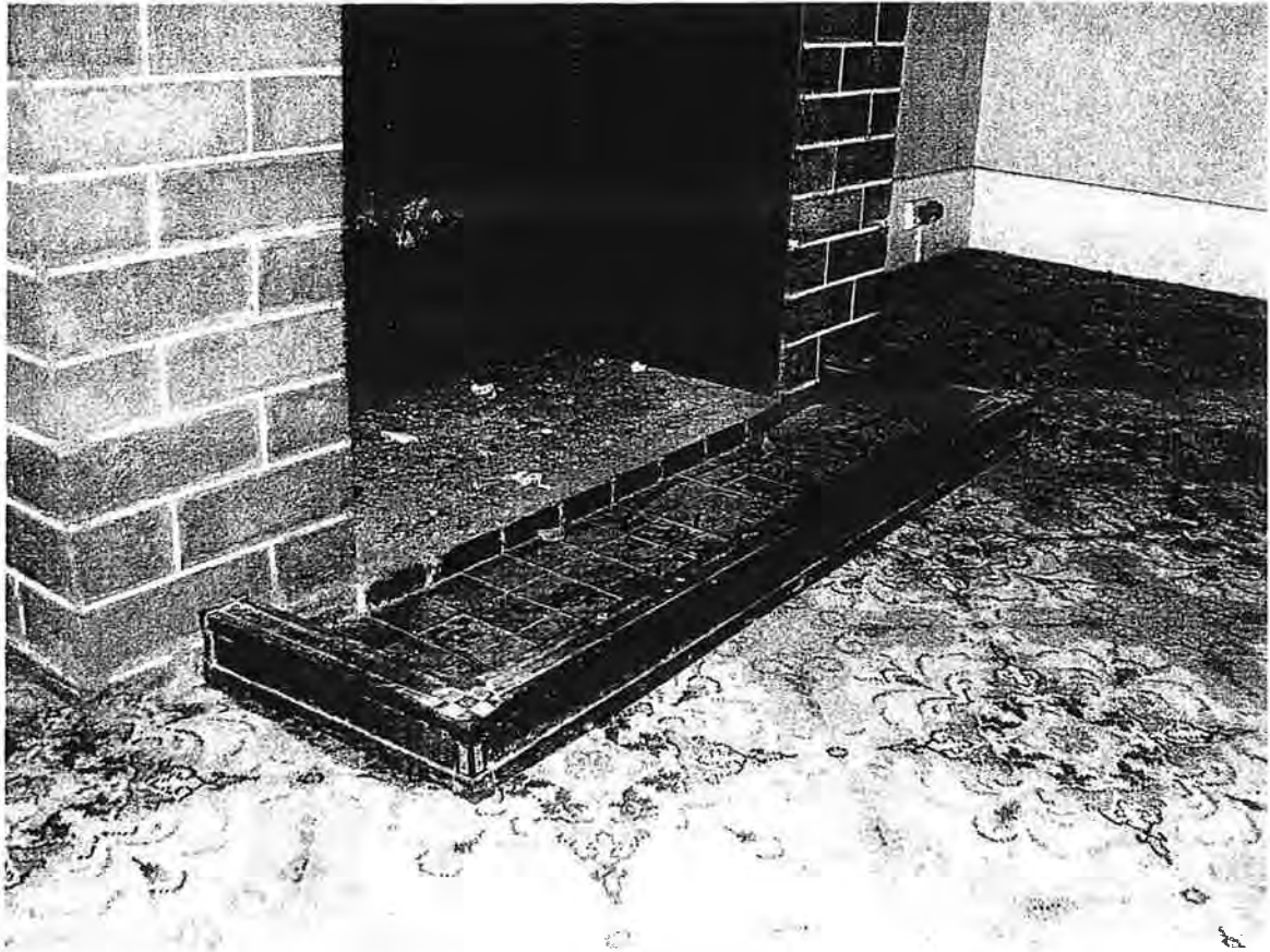
Dining Room Fireplace & Hearth Copper Sheathed (over timber) Fireplace Fender
