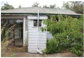
R3 Window Facing N
