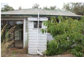
R3 Window Facing N
