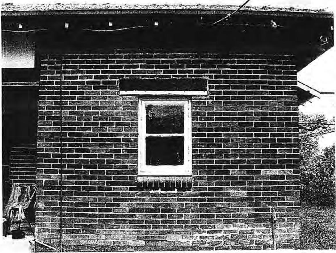
External Window Detail - Rear Bedroom (awning removed)
