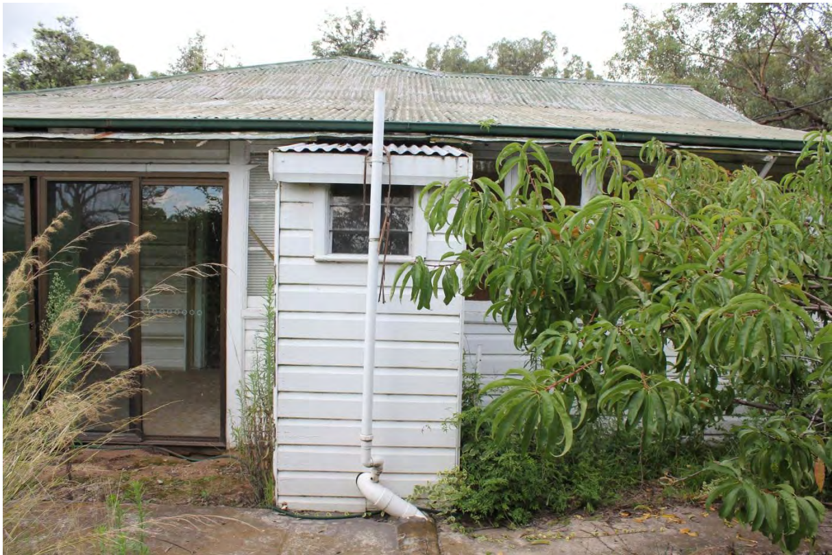
Photo 7: Toilet constructed on western wall of the dwelling.
