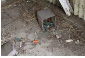
L2 Shed ground
