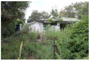
O2 House Facing NW
