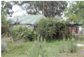
N1 Shed facing NW
