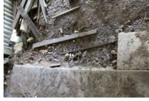
L3 Slab Cut
