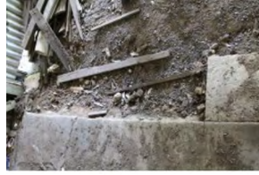
L3 Slab Cut
