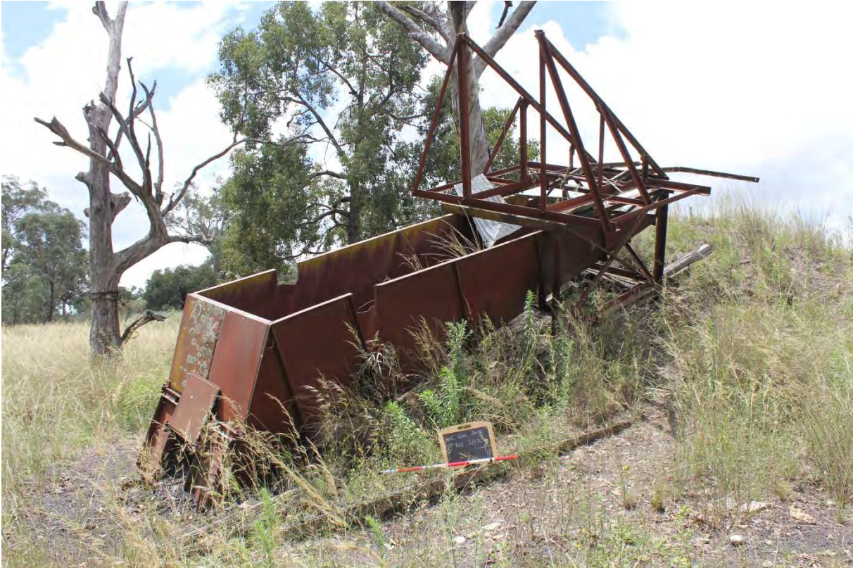
Photo 14: Coal loading ramp and steel chute looking north.
