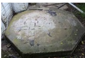
T1 Tank Pad Facing S
