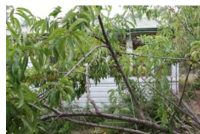
Toilet South Elevation Facing N
