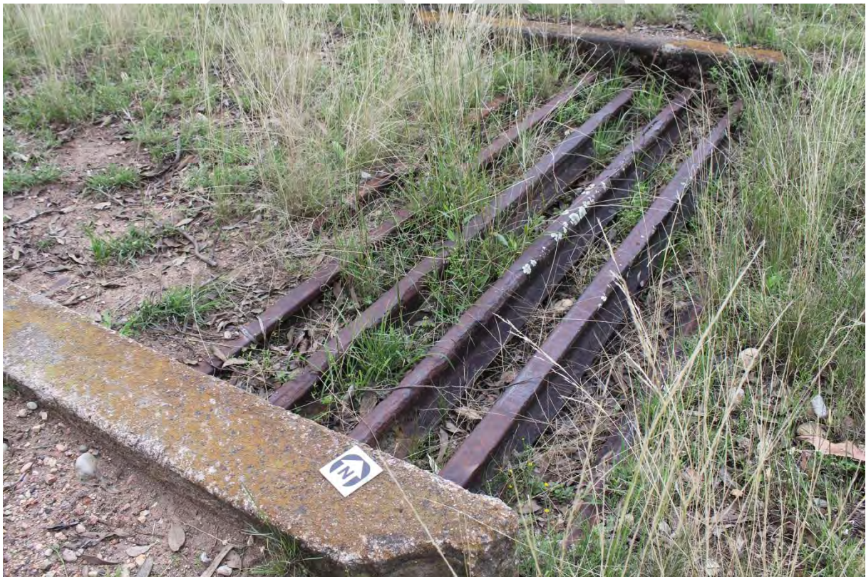
Photo 5: Cattle grid constructed of old railway line located in south western corner.
