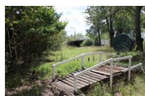
H6 Bridge Facing W
