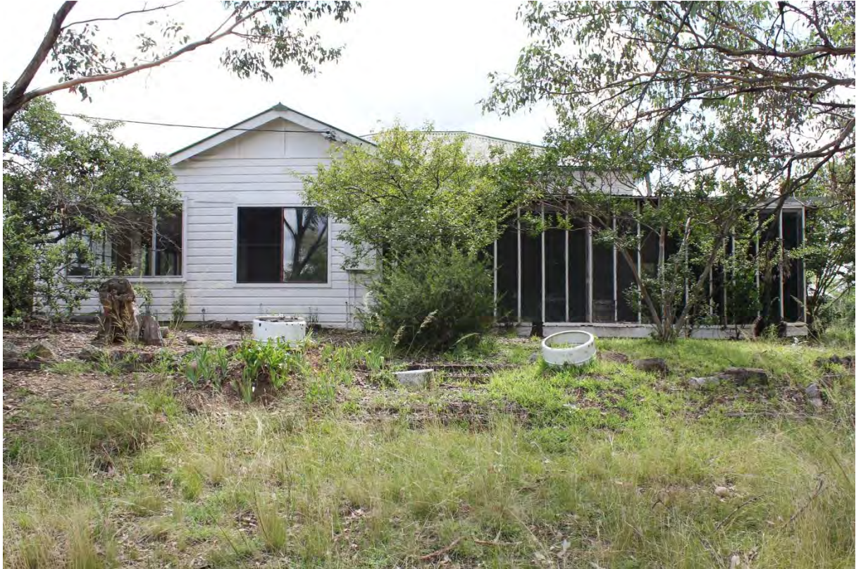
Photo 4: Deputy Mine Managers Residence facing North West.
