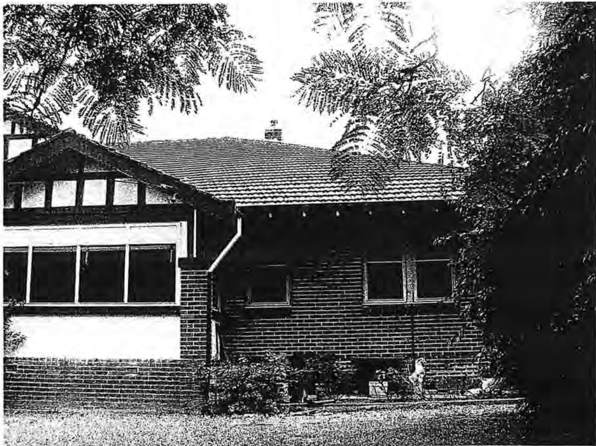
Part of Eastern Elevation
