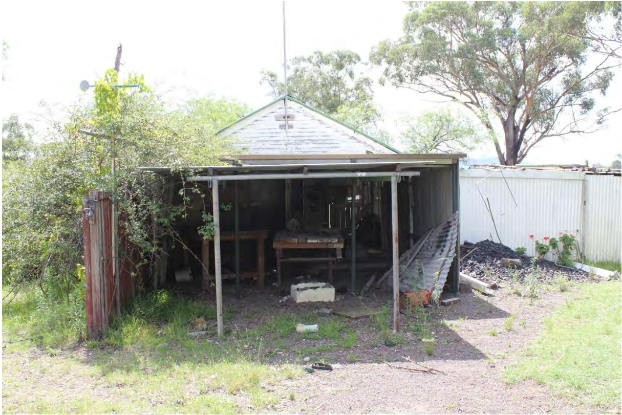
Photo 12: Shed facing west. Note coal stockpile in right of photo.
