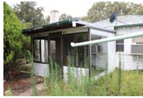
South Elevation Sunroom Facing N
