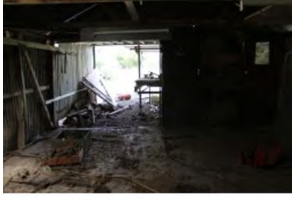
L1 Shed Ground
