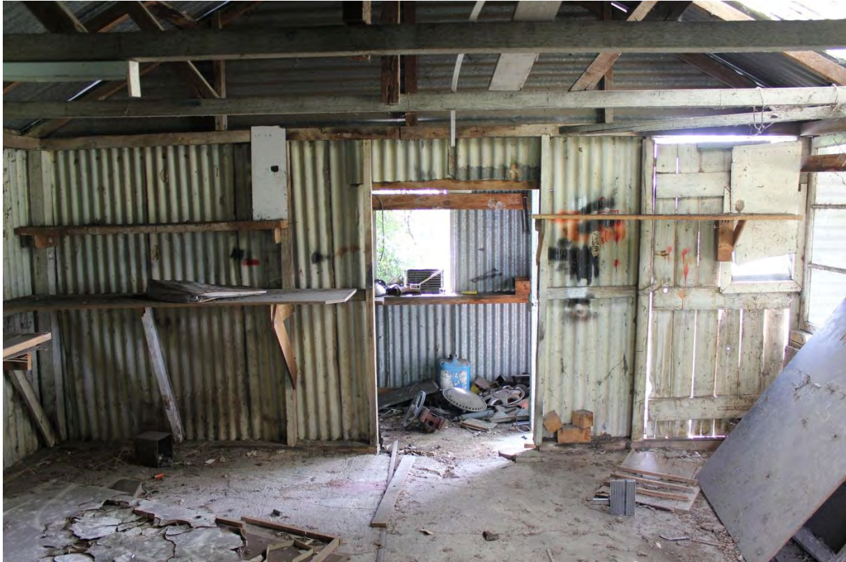
Photo 13: Inside the shed facing west. Note various remaining items.
