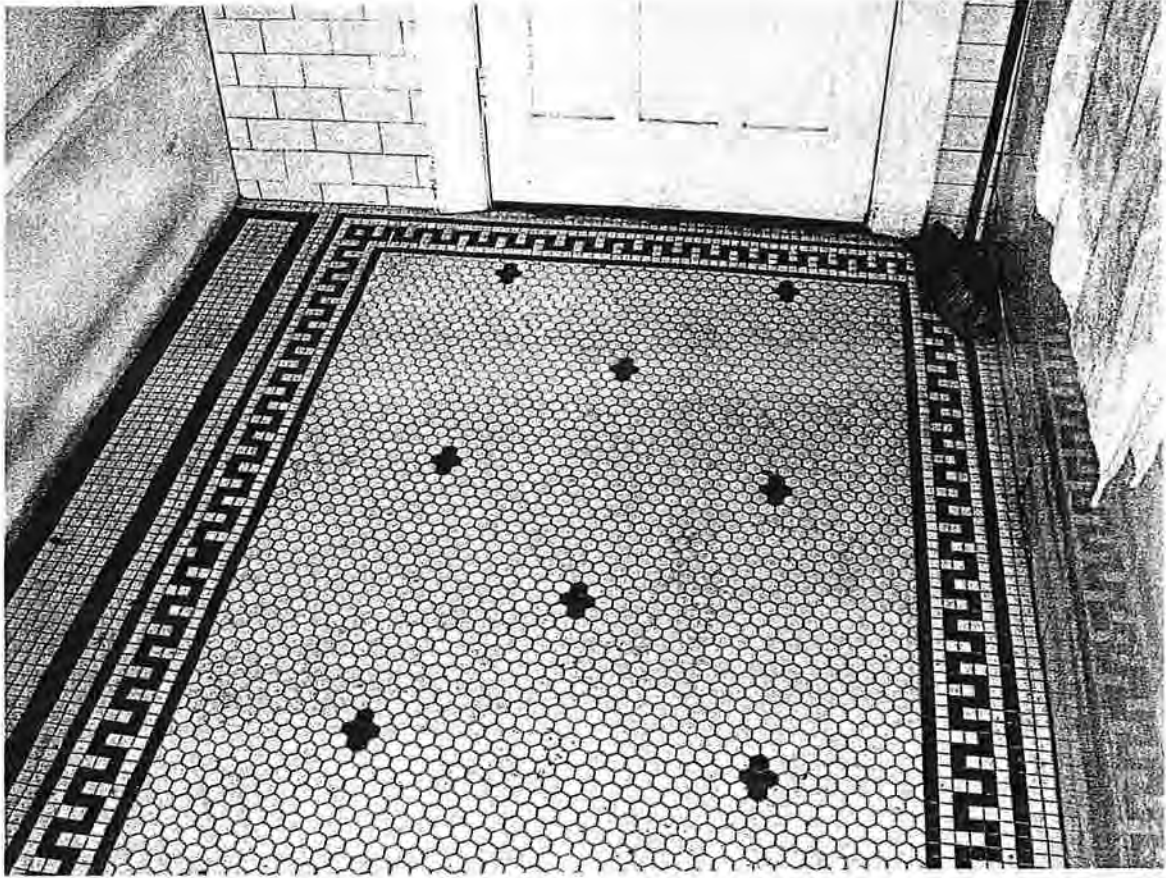
Central Bathroom - Floor Tiles
