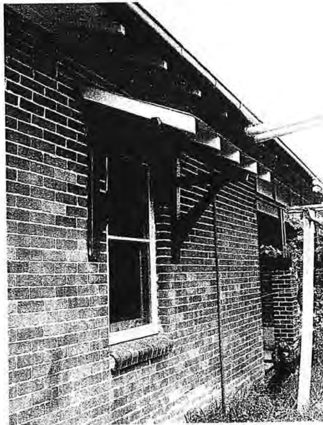
External Window & Canopy Detail - Rear Bedroom
