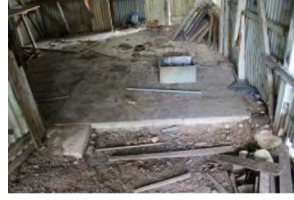
L4 Slab Cut
