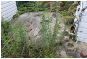
P2 Tank Pad Facing N
