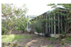
H9 veranda facing S
