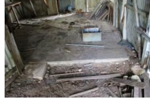
L4 Slab Cut
