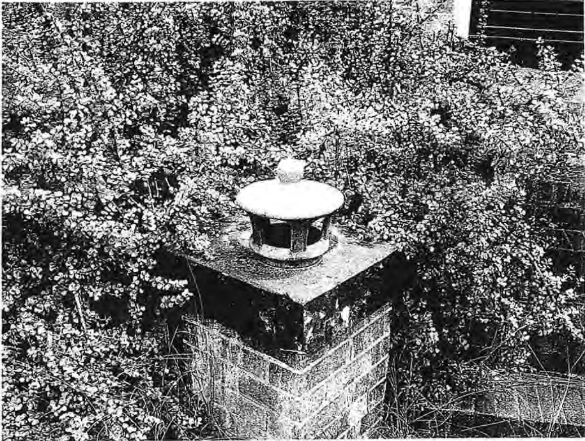
Terra Cotta Chimney Pot (out of place)
