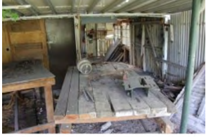
K1 Shed Facing NW
