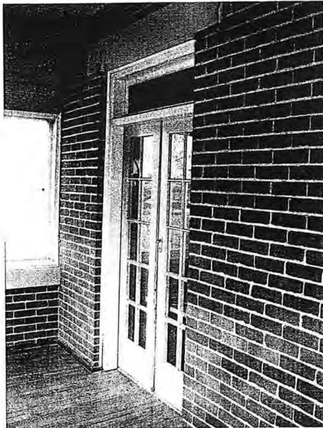
Front Verandah - Doors to Main Bedroom
