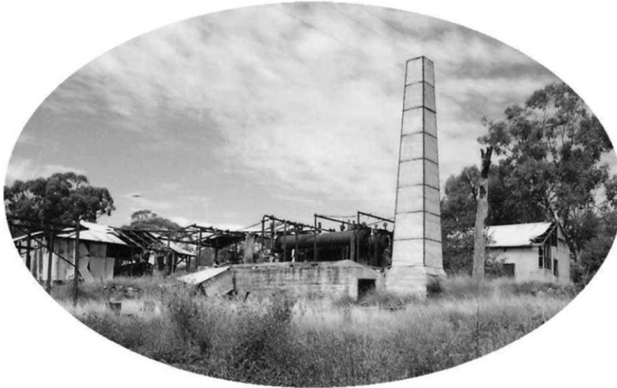
Photo 16: Concrete chimney and former above ground structures circa 1970 (Source: McEvelly et al , 2004 in Landscape, 2005)
